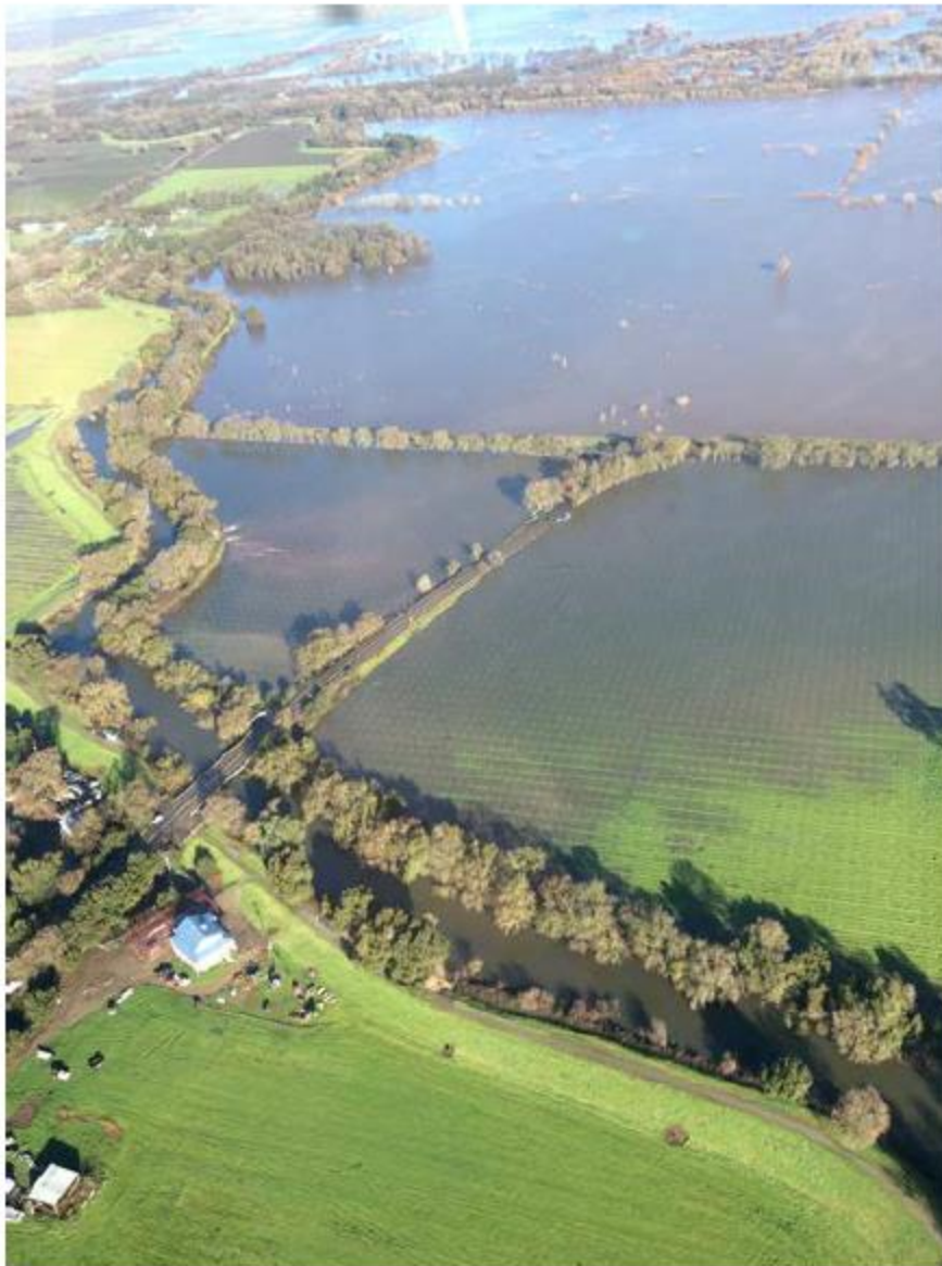
Figure S-12 New Hope Levee Break
