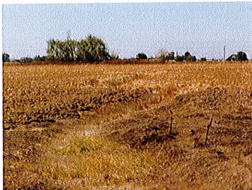
Figure 2.2.4 Florin Creek Channel Downstream of CTRR
