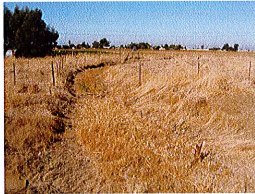
Figure 2.2.5 Florin Creek Channel Downstream of South Watt Avenue
