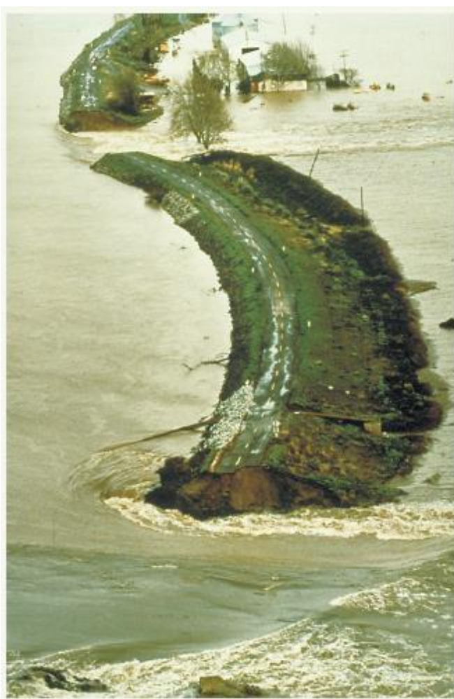
Figure 4-49 1986 Tyler Island Levee Breach
