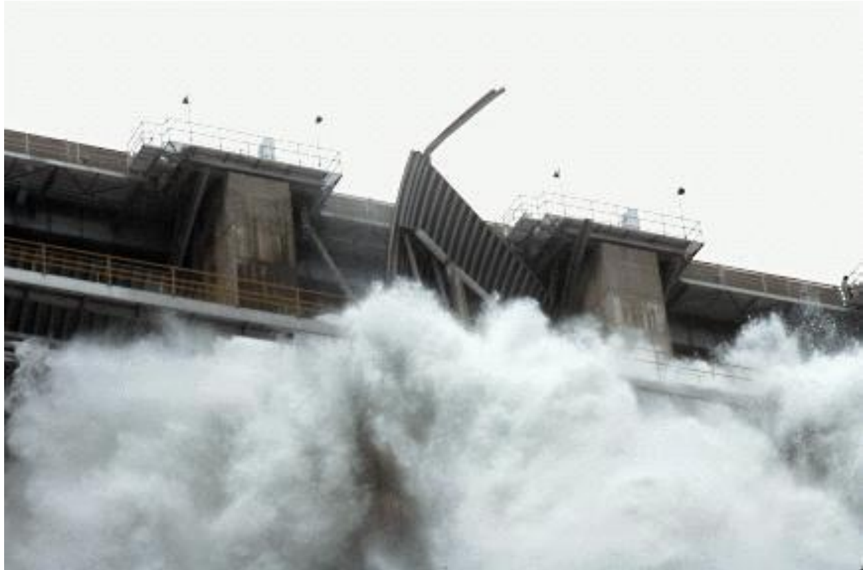
Figure 4-23 July 17, 1995 Folsom Dam Incident
