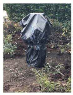
Fire hydrants that are not in service yet, shall be covered with **black plastic bags**. Once the hydrants are in service the plastic bag will be removed.
