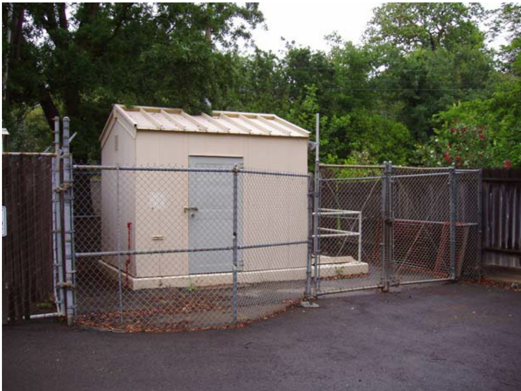
Figure 6 - D-03 Evergreen Estates Pump House
