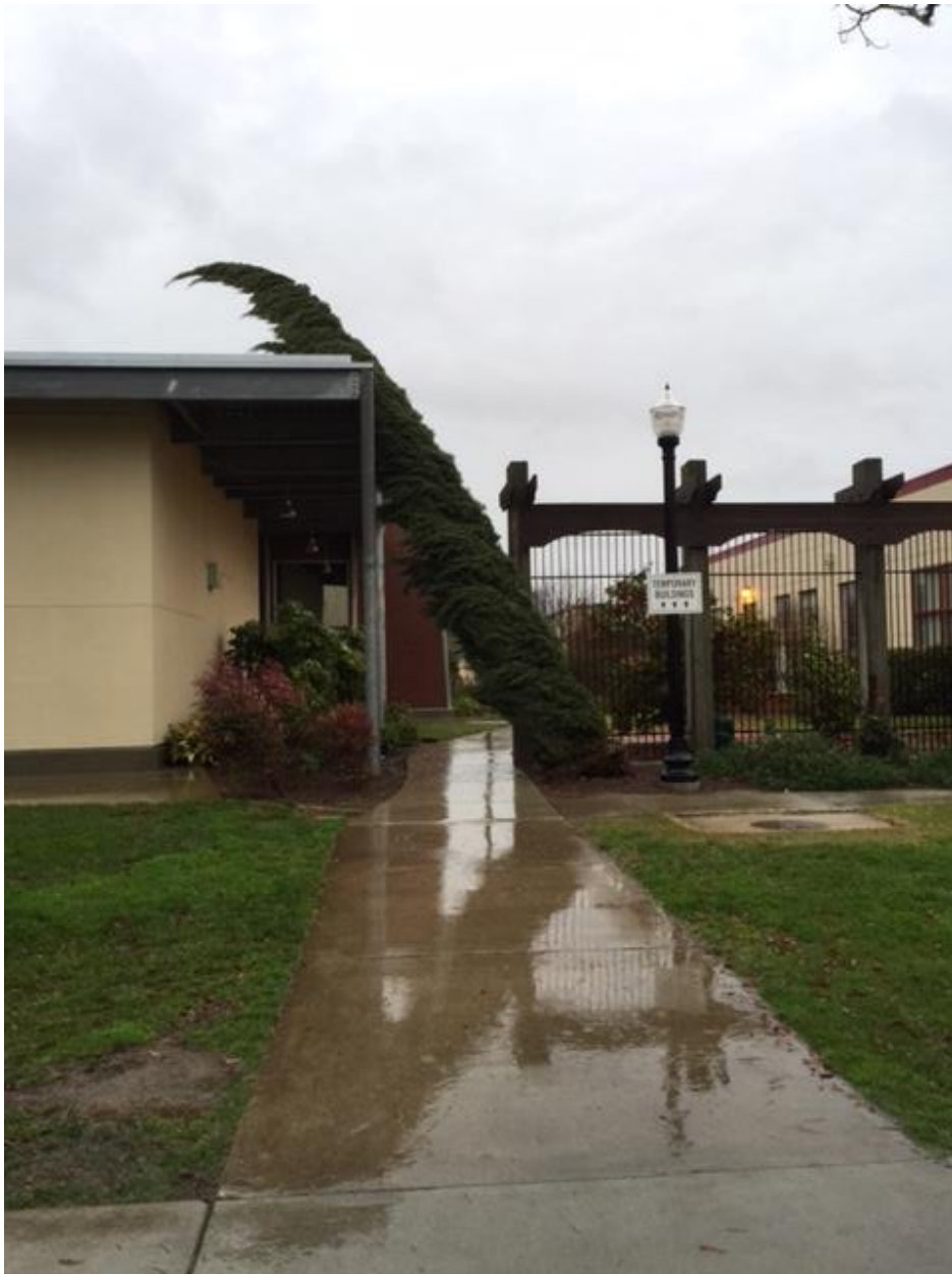
Figure J-5 January 2017 Storm Damage – Felled Tree
