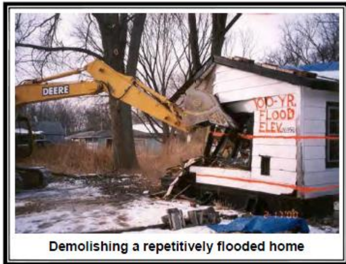
Figure C-5 Demolition of Flooded Home
